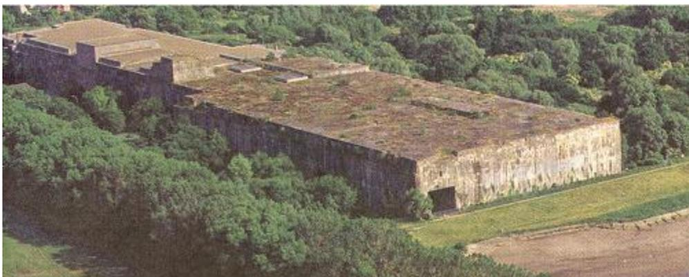
The cavernous interior of the bunker was designed to shelter a production line that could accommodate up to 12 submarines at various stages of assembly. The plan was to bring prefabricated sections of submarines by barge to the facility for final assembly and tests.
